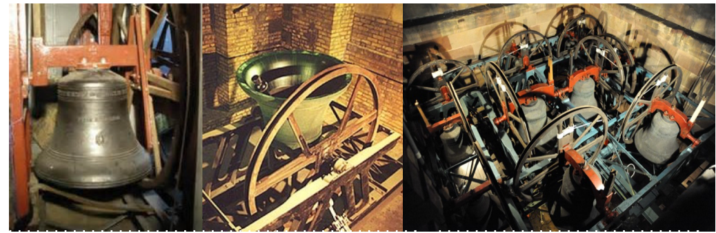
Bell down – can be chimed Bell up – ready for ringing
